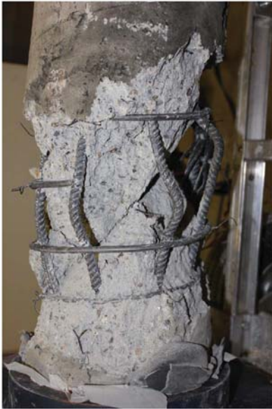
Fig. 13. Failure of the RC column under axial loading due to a shear crack initiated under blast loading (image by Arash E. Zaghi)
