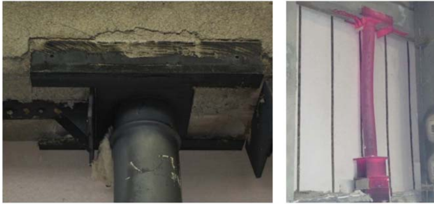
Fig. 11. Local and global buckling of specimen columns tested in fire (images by Michel Bruneau)
